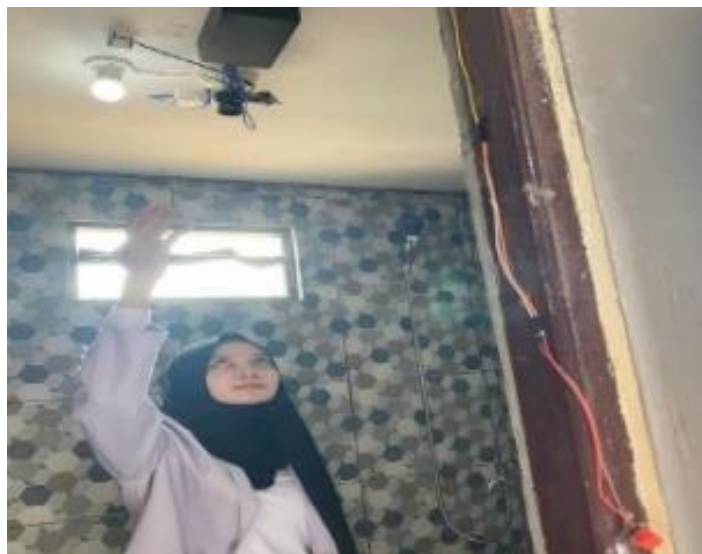
Figure 2: Aerial View of the Toilet's Equipment
